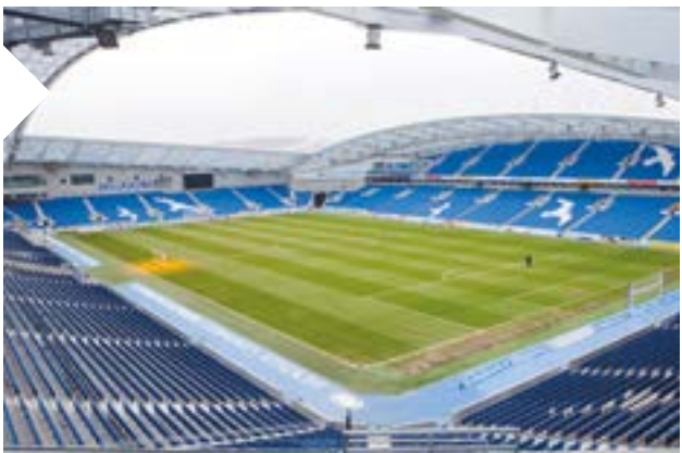
Stadium 8 Atlas Traction MRL lifts, 1 FlexyLIFT, American Express Brighton Stadium, UK
