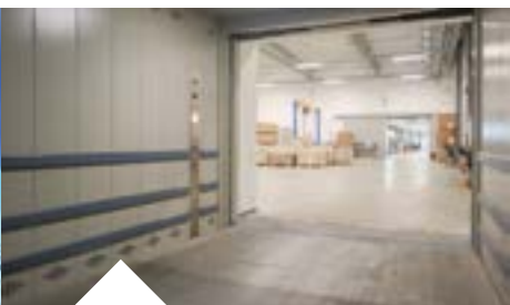
Manufacturing Facility Hydraulic Goods Lift (rated load 13.500 kg) & FlexyLIFT, Sefar, Romania
