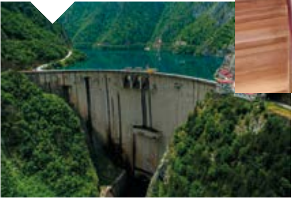
Dam Traction Passenger Lift, Mratinje Piva, Montenegro
