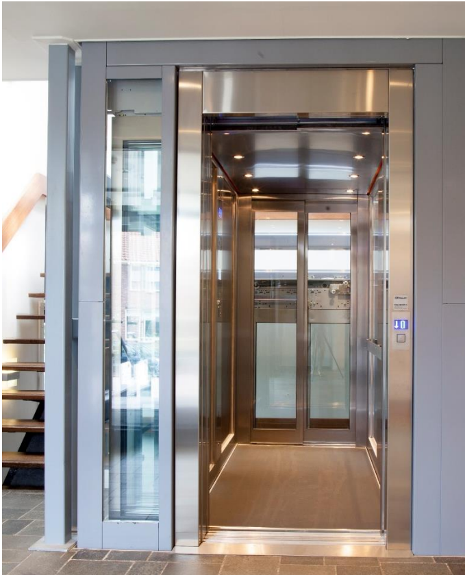
Hospital medical center Baarn, Netherlands
