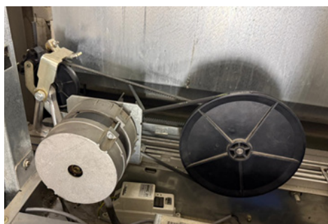
Car Door Mechanism
