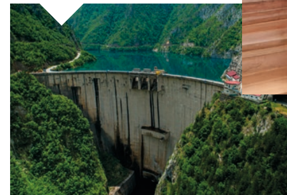
Dam Traction Passenger Lift, Mratinje Piva, Montenegro
